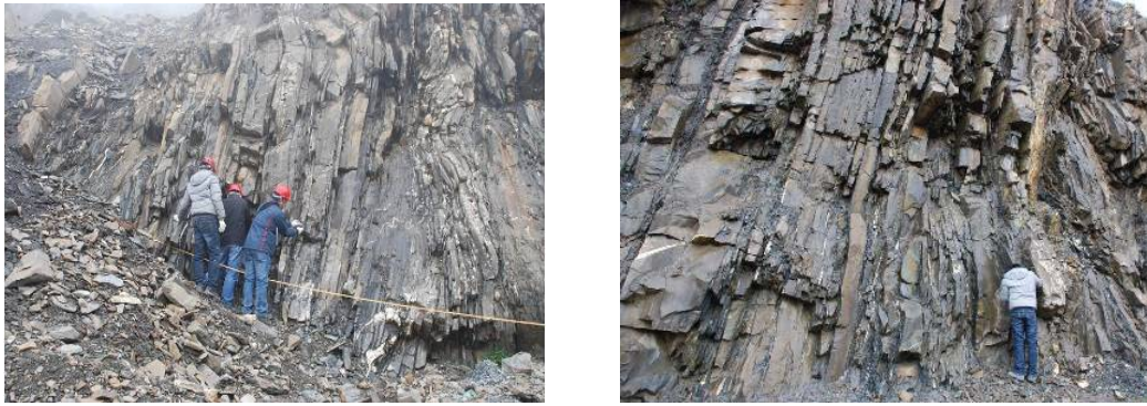
Figure1 An overview of the joints in tunnel site
